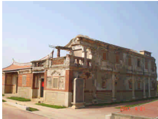
Figure4. Left side of the Bei-shan Mansion has been rebuilt.
